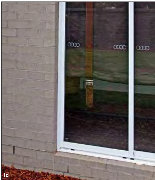
Figure 6 Articulation joints at window/door openings
